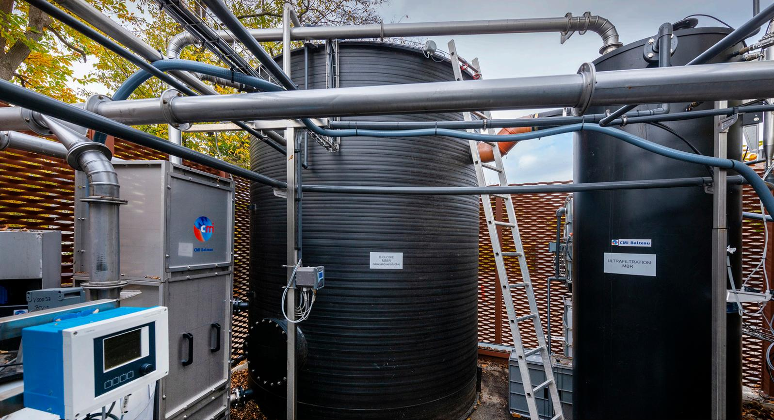
The first step in the process involves promoting the development of microorganisms that can degrade micropollutants in a bioreactor divided into ecological 'niches'. These microorganisms take the forms of flocks (suspended in the bioreactor) and colonies (fixed to synthetic materials suspended in the bioreactor by aeration) called 'biofilms'. They evolve alternatively under aerobic (with dissolved oxygen) and anoxic (without dissolved oxygen but with nitrates) conditions.
